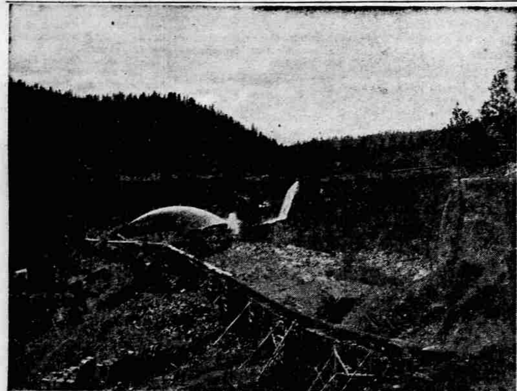
STERLING MINE - This picture of work at the famous Sterling mine, one of the most productive in the Applegate area during the gold mining period at the turn of the century, was taken about 1900. The Applegate valley area spotted with mines which no longer are productive.
