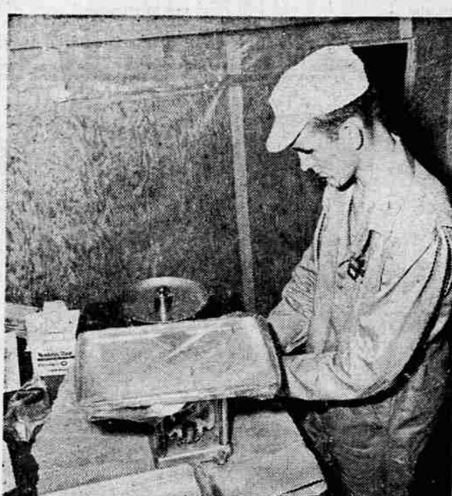
CHECKS FALLOUT —Charles B. Bennett, nephew of Mr. and Mrs. C. C. Vandagriff, 1564 South Whitman ave., Medford, measures the deposited synthetic fallout of radionuclide lanthanum 140 at the Naval Radiological Defense Laboratory in San Francisco. He is majoring in engineering at Stanford university, and was assigned by the laboratory to participate in a field operation at Camp Stoneman. He is a member of the National Merit Scholarship program.
