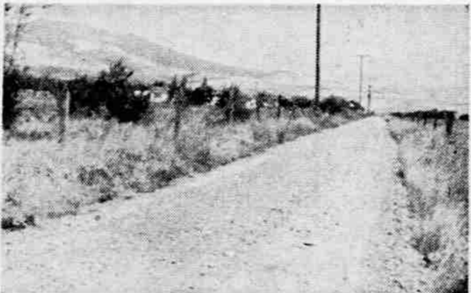
NARROW ROADWAY —This road measures 16 feet in width between fences making it difficult if not impossible for two cars to pass. The road serves eight houses. The road dead-ends with no turn-around provided.
