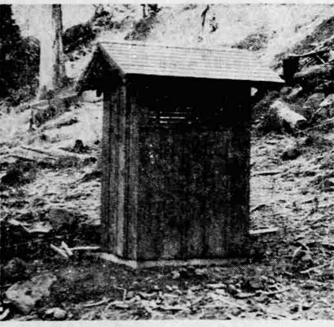
NEW TYPE - The rest room above, recently erected at McCallister soda springs camp site is the new type being put into use by the Forest Service. The pre-fabricated building features a concrete slab floor and other sanitary features. Trees will be planted throughout the camp area that will, in a few years, provide shade and privacy.
