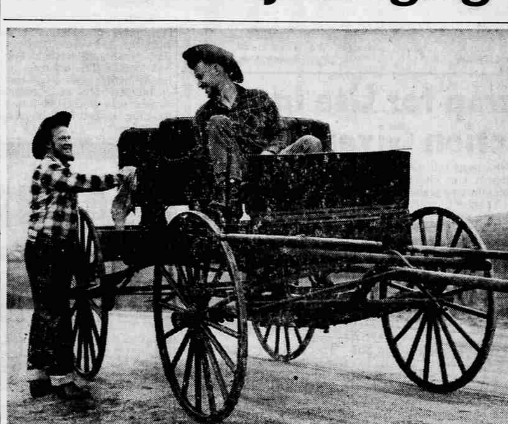
SURREYS READIED - Visitors in Jacksonville will soon have the opportunity to take a real old-fashioned "buggy ride" when partners Lee Garland and Dave Taylor finish renovation of two surreys to use in their guided tour service of the historic town. The men have acquired the franchise to operate the horse-drawn vehicles in connection with Oregon's centennial celebration.
