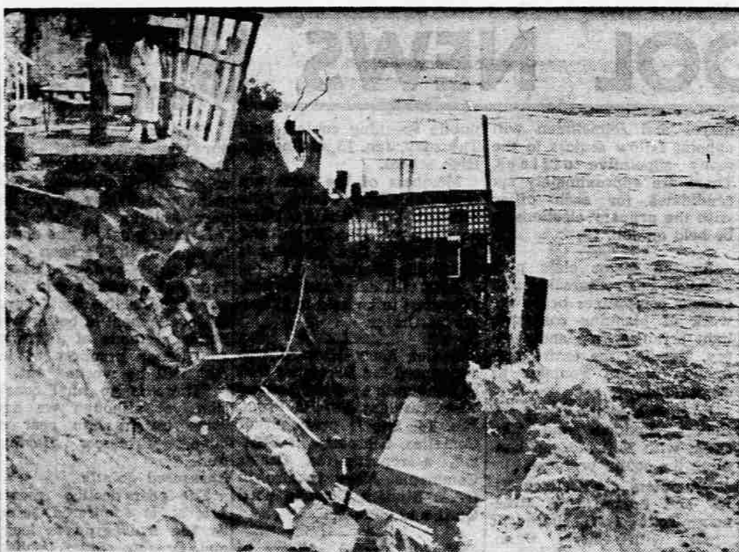
HIGH TIDE DAMAGE —The home of Bob McGraw on the Pacific Coast in Malibu, Calif., is imperiled by erosion caused by unusually high tides which have caused much damage in the area. Patio and ping-pong table are already gone, and the waves keep coming in.
