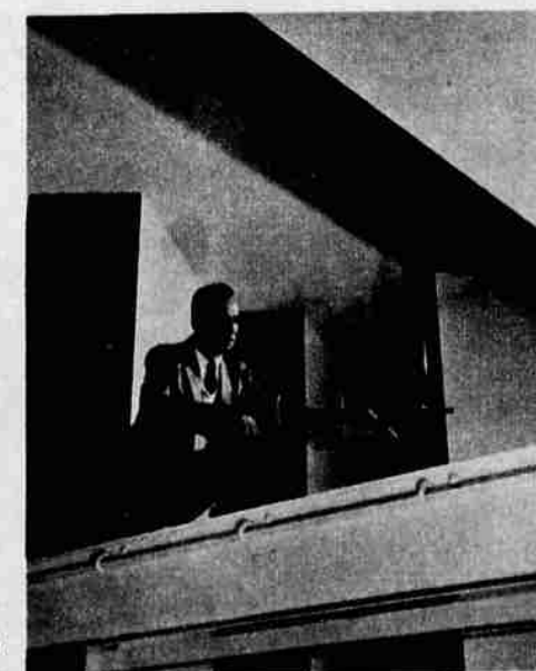
Dr. Robert Benson, Armour Research physicist, adjusts microphone in reverberation chamber to test jet engine noises.
