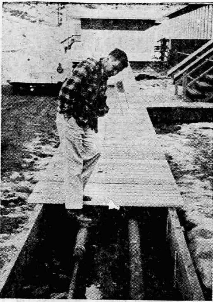
SNOW PROBLEM —Newsman Al Cocking, visiting Squaw Valley, Calif., scene of the 1960 Olympic Winter Games, inspects steeply pitched roof under board sidewalk to melt snow and eliminate the back-breaking job of shoveling the walks. Presently this is no problem as the area, like most of Northern California, is experiencing the worst drought since the days of the Gold Rush.
