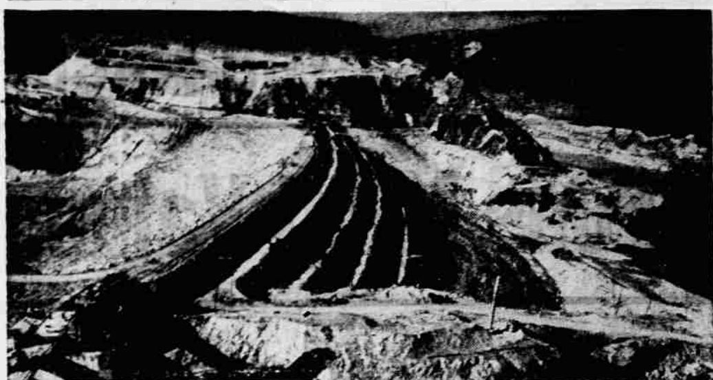
BACKING UP WATER from Lewis River and Swift Creek, Swift Dam, world's highest earth-filled dam, 512 feet, has been completed at Cougar, Wash. Power generation and transmission installations now are being completed. Dam cost $56,000,000.
