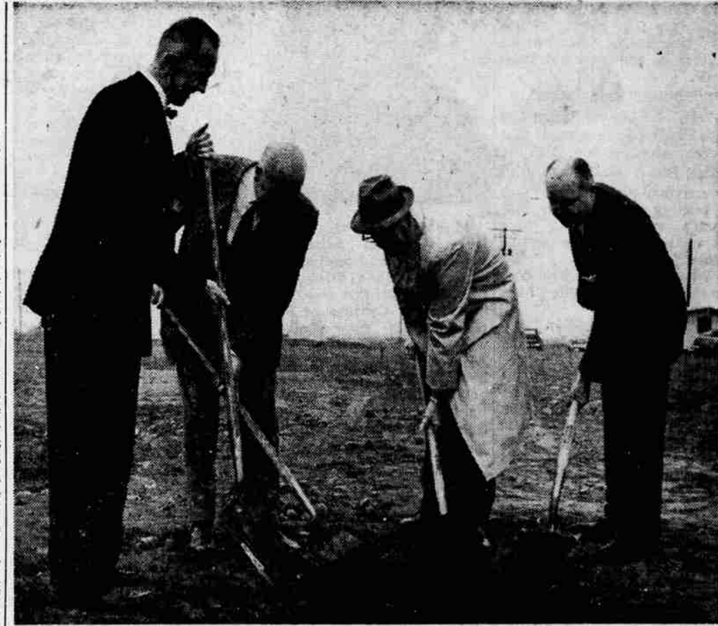
SPADEWORK—"Breaking ground" at the site of the Sears Roebuck and company store in the proposed East Jackson st. shopping center yesterday are Otto Frohnmayer, president of the Jackson County Chamber of Commerce; Mark Goldy, local agent for the center's developers; Medford Mayor John W. Snider and W. Price Sullivan, northwest zone manager for Sears.
