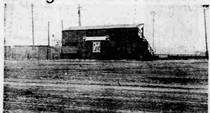
POSITIVE STEP —Recognize this scene? Seen anything different? Cheney Forest Products of Central Point has cleared out the weeds and leveled the ground. According to Bill Askwith, Cheney's manager, the grandstand is to be painted next spring when the weather is suitable. Kogak Lumber Industries has also done extensive clearing work to the south. Starting today, the Mail Tribune's inventory includes pictures of "Making Medford Beautiful" as well as those of eyesore that still exist.
