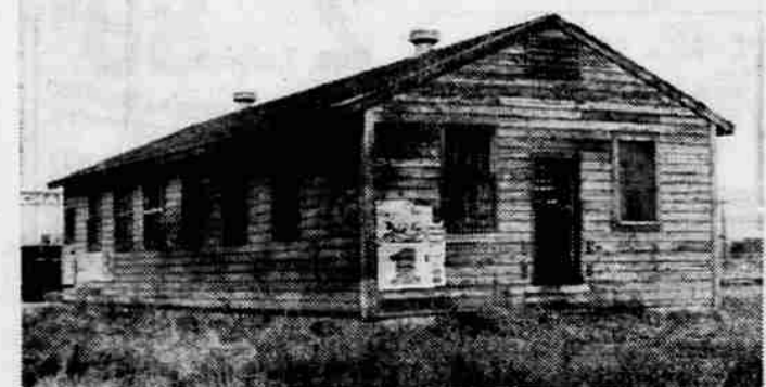
ABANDONED —This orphan of an apparently neglectful property owner stands beside one of Medford's busier streets. Its windows are broken, its walls unpainted, its immediate surroundings choked with weeds. The only bright spots are well-weathered carnival posters. Demolishing or rehabilitating such structures can contribute greatly to "Making Medford Beautiful."
