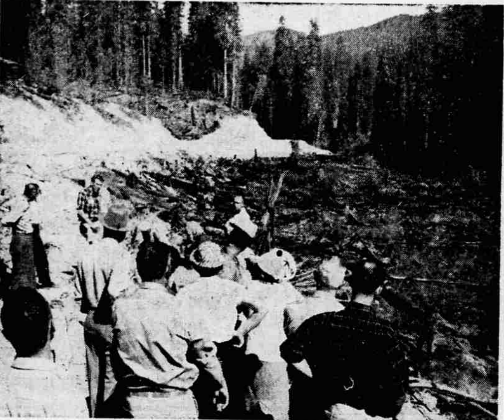
CLEAR CUT —The sight presented by a logging operation that has denuded whole blocks of forest land is not a pretty one, with charred logs lying helter-skelter where green trees once stood. With natural reproduction or replanting the scar soon heals and a new forest begins to rise above the clutter. Some sections of the road leading to this area, in the Flat creek section, cost $25,000 per mile to build.
