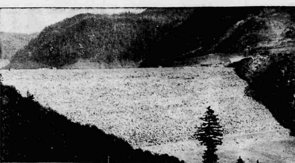
CLOSING DIVERSION TUNNELS , engineers start filling world's highest earth-filled dam, at Cougar, Wash. It measures 475 feet in height. Runoff of Lewis River and Swift Creek from sides of Mt. Adams is expected to fill dam by December, when power generating facilities are installed and dam is put "on line" providing industrial power.
