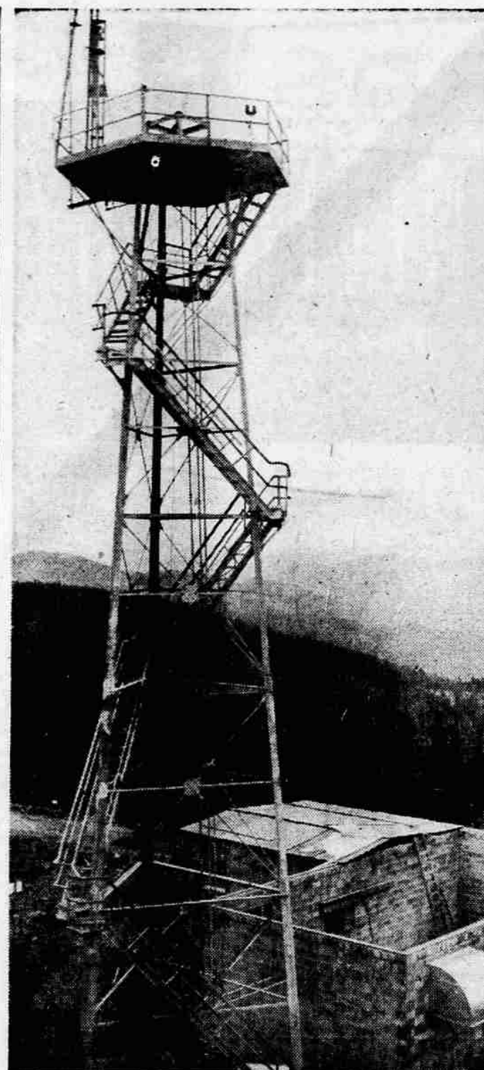
"GAP FILLER" STATION—Placer Air Force station, located atop King mountain near where the Josephine, Jackson and Douglas county lines come together, is nearing completion. The picture above, taken from the state department of forestry lookout also located on King mountain, shows the nearly-completed tower, and the as-yet roofless buildings of the radar station, which is a "gap filler" facility, to close up a "blind spot" in the Pacific Coast's radar network. Construction of the station, delayed by the construction and transportation labor disputes, is due for completion in a few weeks. The view above is looking toward the northeast.
