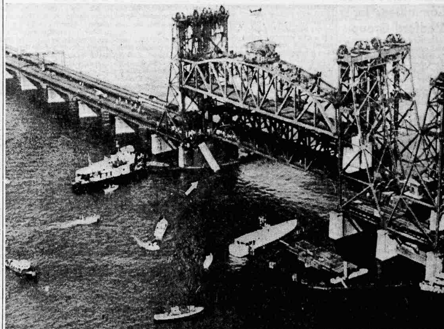
COMMUTER TRAIN DISASTER —General view shows the drawbridge at Bayonne, N.J., where two locomotives and three passenger coaches of a New Jersey commuter train ran through an open drawbridge and plunged into the water of Newark bay. Note near side of the drawbridge, raised up above the tracks. One of the coaches can be seen (arrow, center) still hanging from the open end of the bridge.
