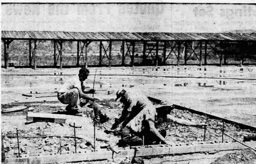
WORK ON RIFLE CLUB BUILDING—
