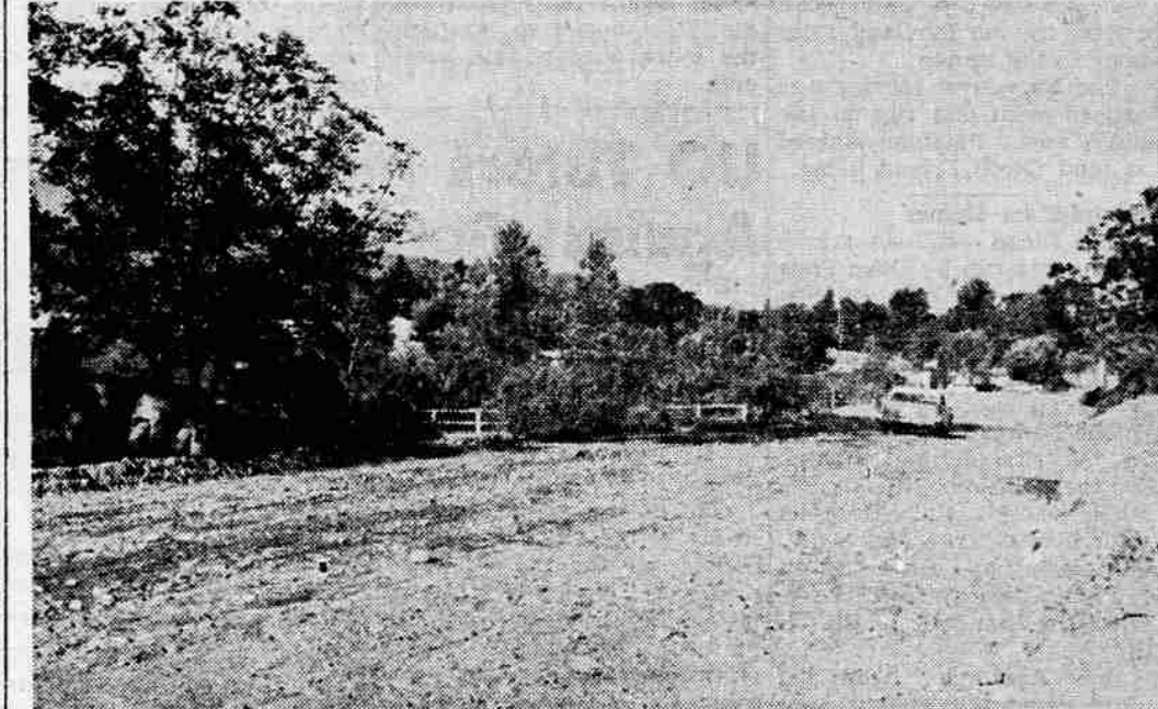
JACKSON STREET EXTENSION — Excavation work for the extension between Barneburg rd. and Sunrise ave. has been completed. Next comes installation of base material, leveling and paving. The street was open temporarily to traffic last week, but few motorists braved the bumps.
