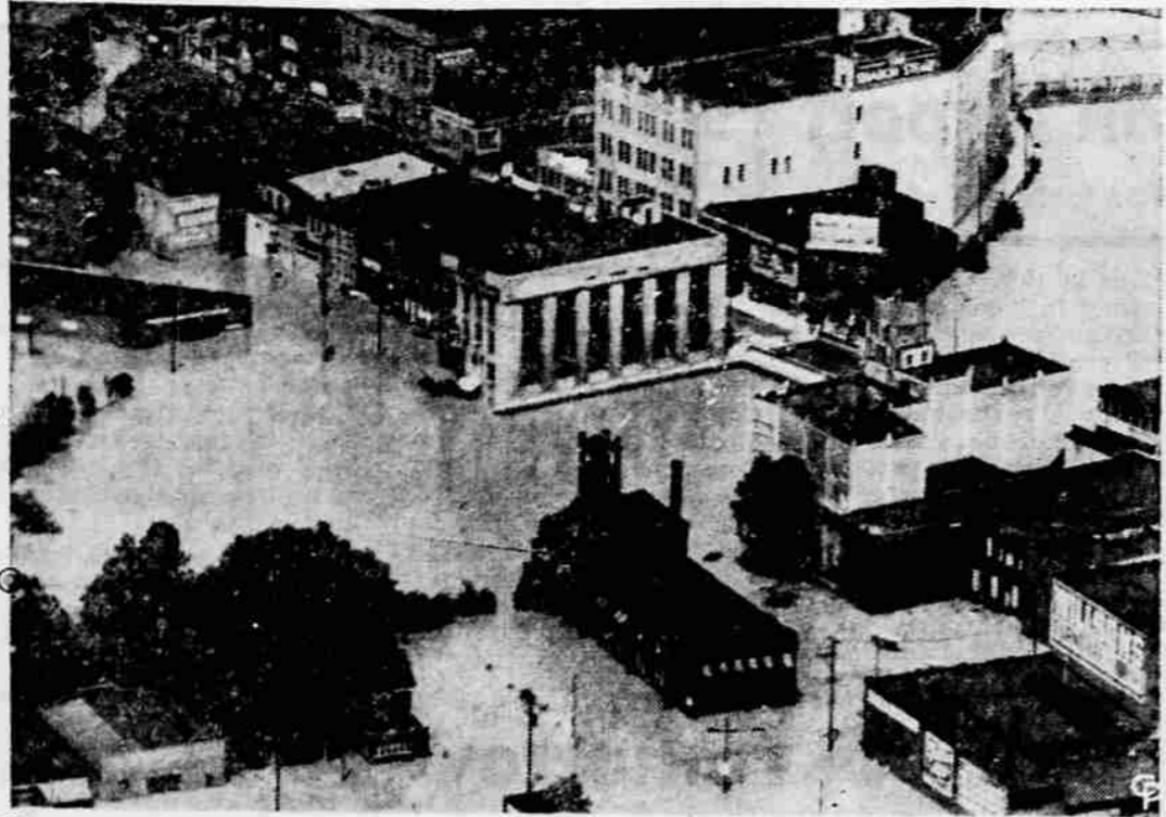
BURYING SHAROM, PA. , under many feet of water, worst flood since 1913 forces thousands to seek higher ground, causes damage running into millions of dollars.
