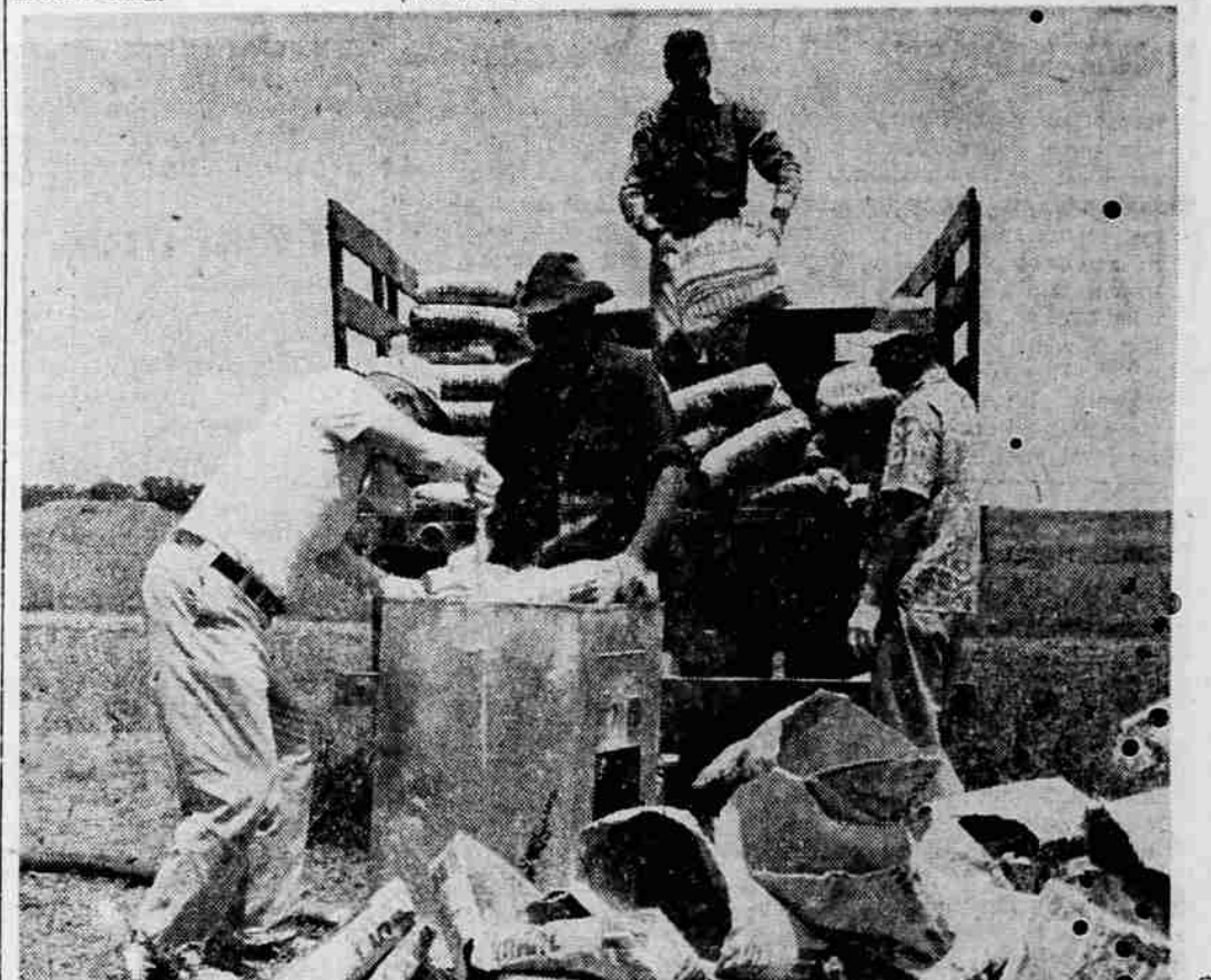
CHECKS CONSISTENCY — T. S. (Tenny) Moore, (above) fire control officer of the Rogue River National forest, tests the consistency of the chemical fire control slurry as it comes out of the discharge pipe below the storage tank. Special tanks on Medford Air Service planes will be filled by gravity flow from this outlet. This type of chemical fire control has never been used before in this area, according to Moore.
