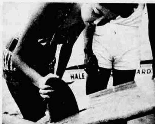
3 Short keel under rear end of surfboard gives it some stability. Remainder is furnished by the agility of its rider.
