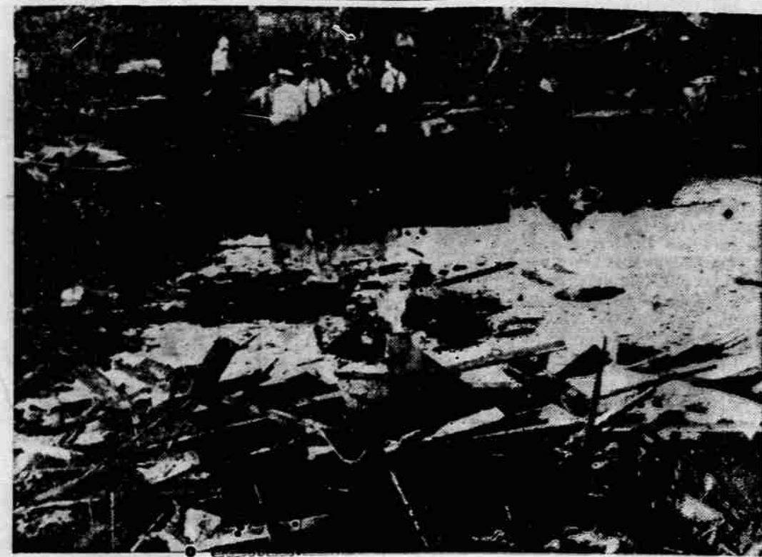
FIREWORKS BLAST KILLED ONE — Fire and shattered windows as far as 22 blocks inspectors (background) examine scene of explosion in Portland, which razed nearby homes on page 3A, second section.
