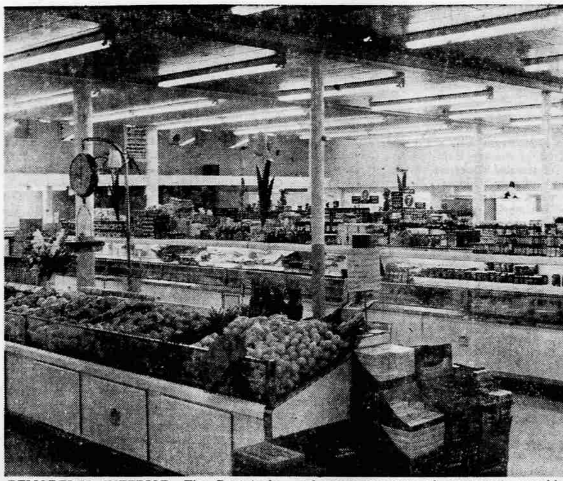
REMODELED INTERIOR —The Groceteria and rearrangements of counters to provide Super market, Grape and Sixth sts., Medford, recently completed a major phase of remodeling which included new lighting offices and a third floor for storage space.
