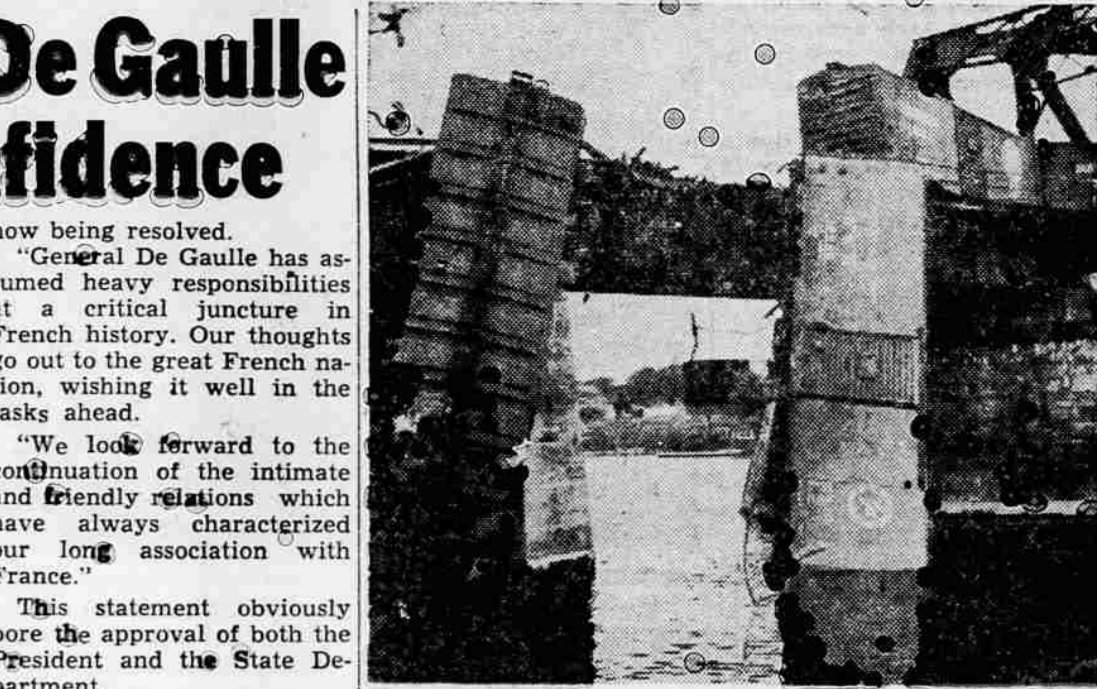
OVER THE SIDE —Two cars of Delaware and Hudson freight train hang over the side of bridge across the Mohawk River at Schenectady, N. Y., disrupting rail and canal traffic. A broken journal on the 99-car train was blamed for the 18-car derailment. Damage to bridge and rolling stock was estimated at $500,000.
