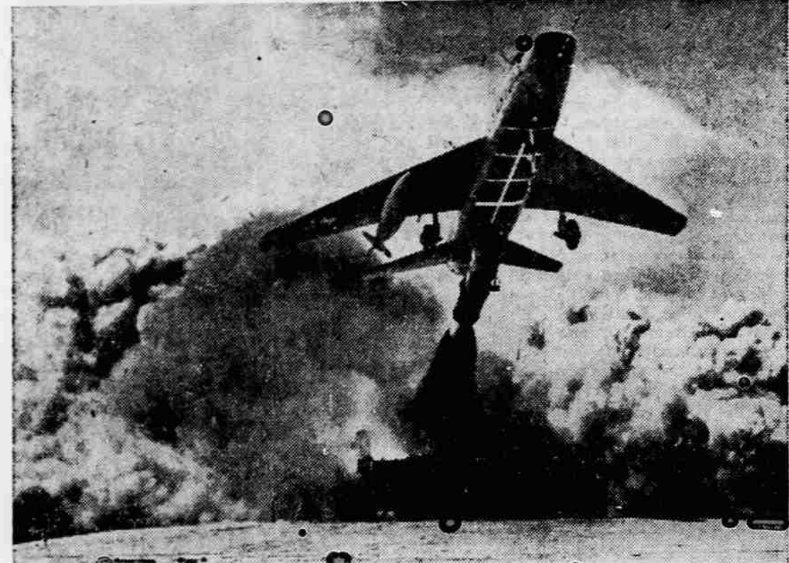
SWOOSH — Air Force F-100D jet fighter leaps from zero-length launcher with the aid of a 130,000 pound thrust rocket booster developed by Astrodyne, Inc., of McGregor, Tex. It was the first successful launching of a supersonic jet plane without benefit of a runway.
