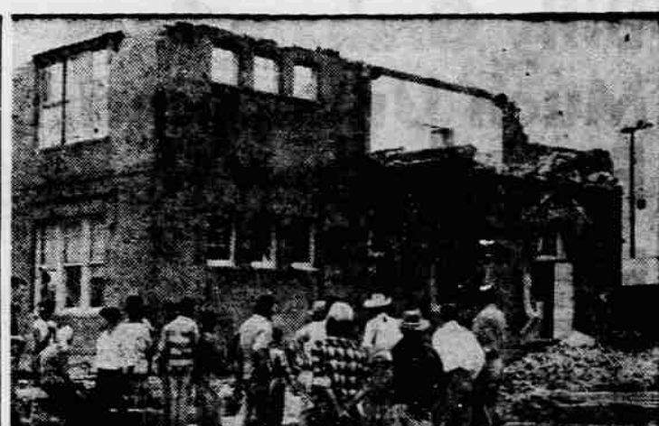
RIPPING ROOF off this school house in LaCoste, Tex., near San Antonio, a tornado miraculously failed to injure 40 pupils. It wrecked more than score of homes. (International)
