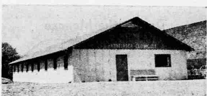
NEW CLUBHOUSE — Medford Pathfinders last week dedicated a new clubhouse at the Rogue River academy grounds on South Stage rd. The building was constructed through work by club members with funds raised from several projects.
