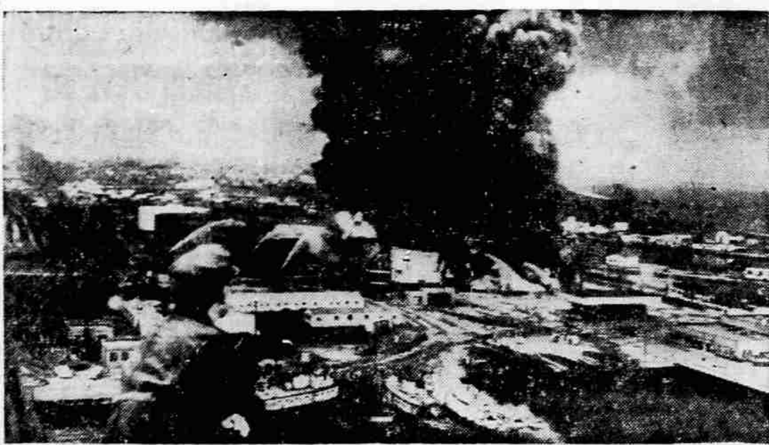
OUT OF CONTROL—Smoke billows storage tanks of Esso Bunker Oil Station in Newport News, Va., where 13 huge tanks have been destroyed. The out of control blaze is believed to have started with an explosion in the plant's control building.
