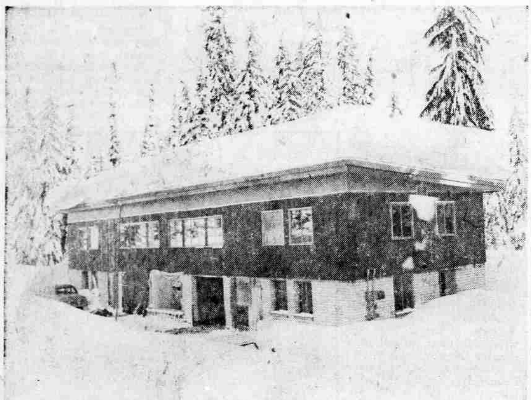
NEW RESIDENCES —Construction started last year on new residences for park personnel at Crater Lake National park near headquarters. Shown above is one of the two-family units, designed to provide living quarters above the average snow level. Roofs are designed to hold the snow pack. Such design, officials said, will eliminate moving snow from around steep roofs so it can slide off.
