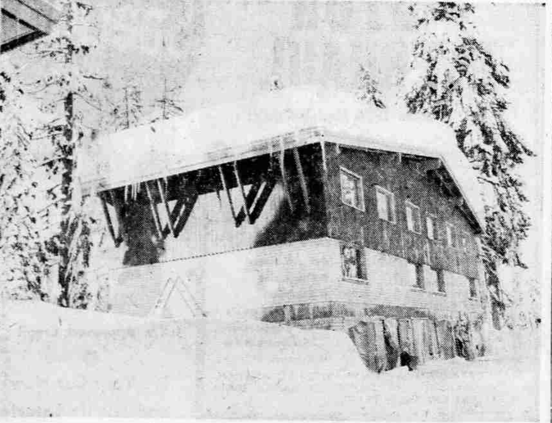
NEW CONSTRUCTION —Part of the Mission 66 program of the national park service is to provide adequate living quarters for park personnel. Above is one of the new four-family units at Crater Lake National
