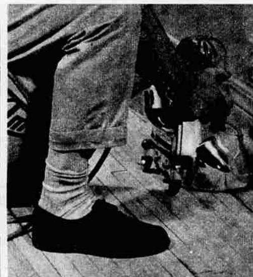
The sander should be used with the grain. Edger does the close work along the sides.
