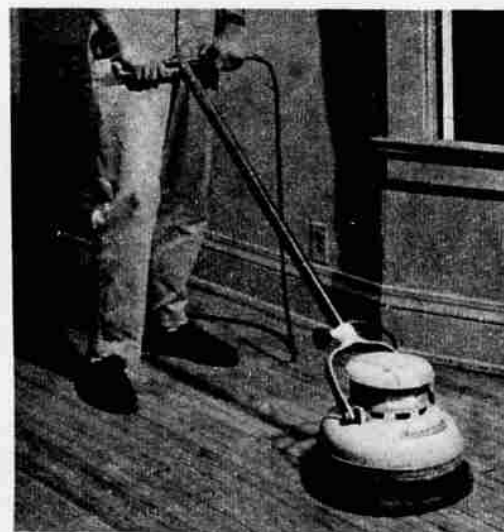
The polisher does the final job with wax.
