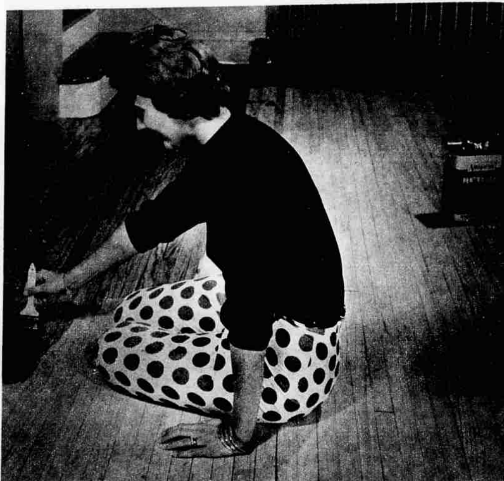
Best protection for newly sanded wood is a penetrating seal that is easy to apply.
