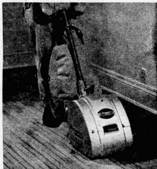
The sander should be used with the grain. Edger does the close work along the sides.
