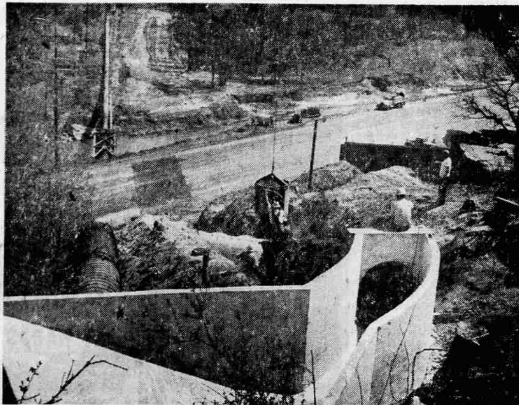
NEARING COMPLETION—Last concrete placement of the Bear Creek Siphon, Talent lateral of the Talent Irrigation district is shown nearing completion. It is located one mile south of Talent and under Bear creek and Highway 99. This
