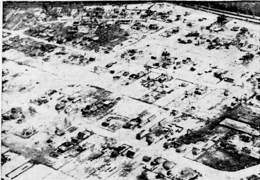
ISOLATING HOMES in Stockton, Calif., flood waters fill streets in San Joaquin Valley city as torrential rains pour water into low-lying areas. (International Soundphoto)
