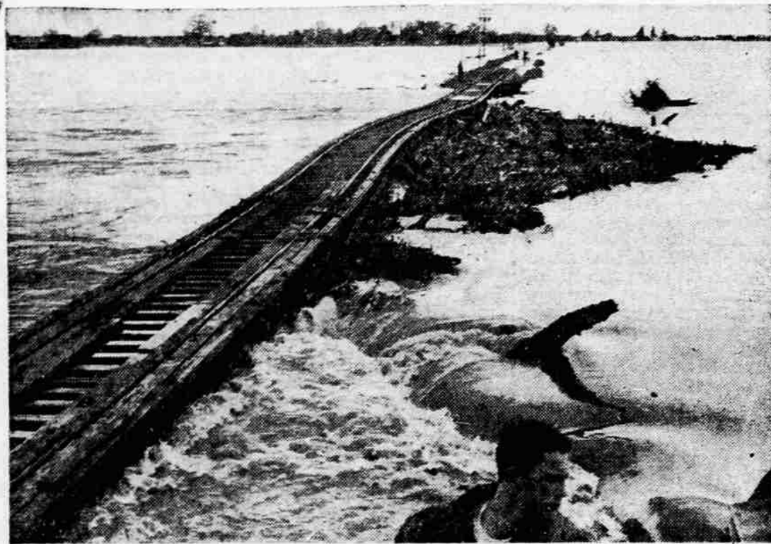
RUSHING WATER—Southern Pacific railroad bridge sags under pressure of debris. Workers in foreground are sandbagging forced against it by the rain-swollen San Joaquin river near Stockton, Calif. Only the rails are holding the span in place. Workers in foreground are sandbagging spot where the road bed cuts through levee.
