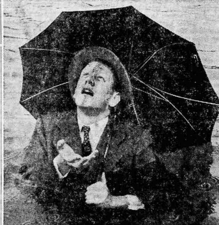
STREET CORNER? —It might well have been any street corner in San Francisco during heavy rains which inundated many sections of the Bay Area. The rains came, and left Bill Zowasky up to his... well, up to here in water. It wasn't really that, but it sure seemed that way.
