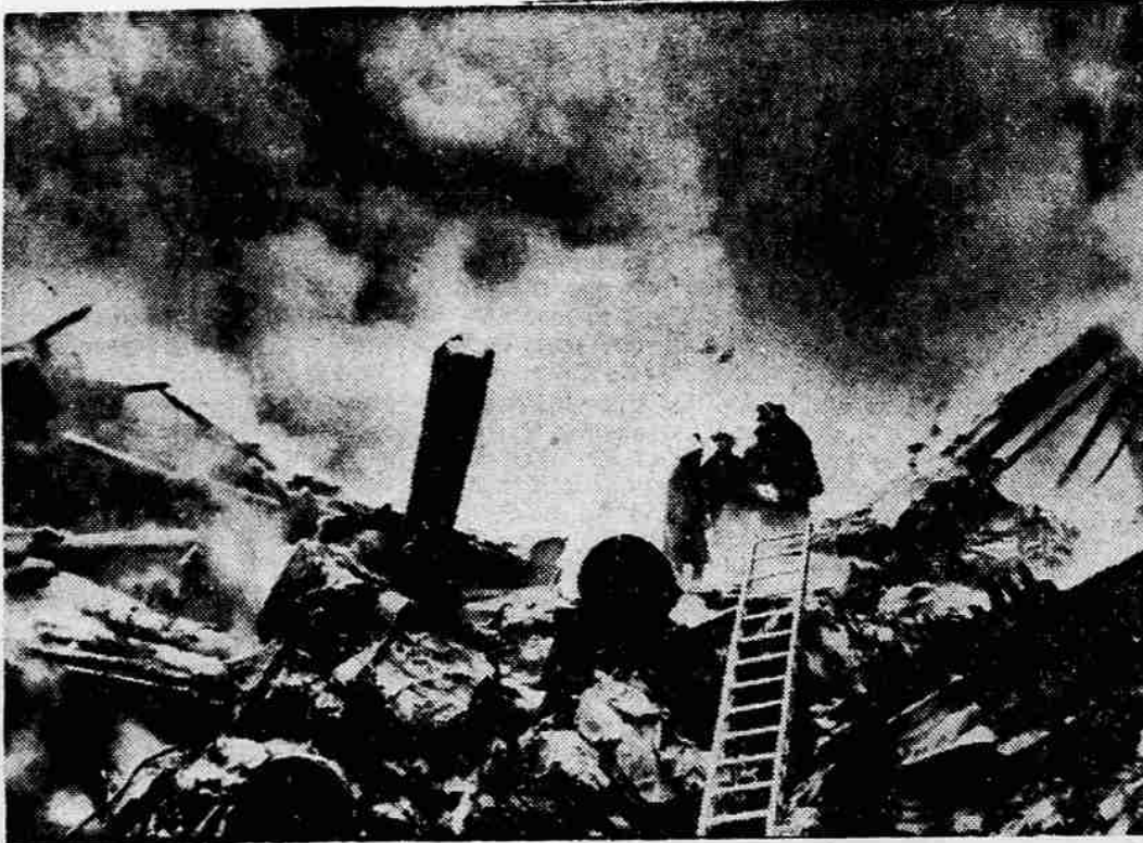
SMOLDERING RUBBLE —Fire chiefs hold conference amid the smoldering ruins of a twine and paper factory which collapsed at the height of a five-alarm blaze in New York. Two firemen were known dead and four others were trapped and presumed dead in the wreckage of the six-story building.
