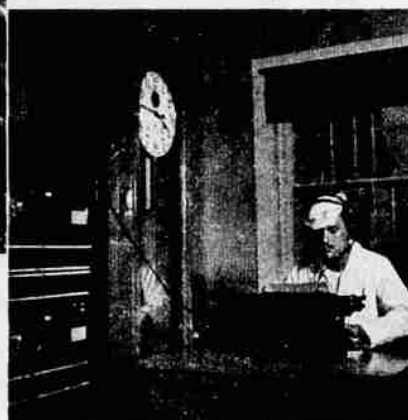
Guardsman winds windlass that makes light revolve.
