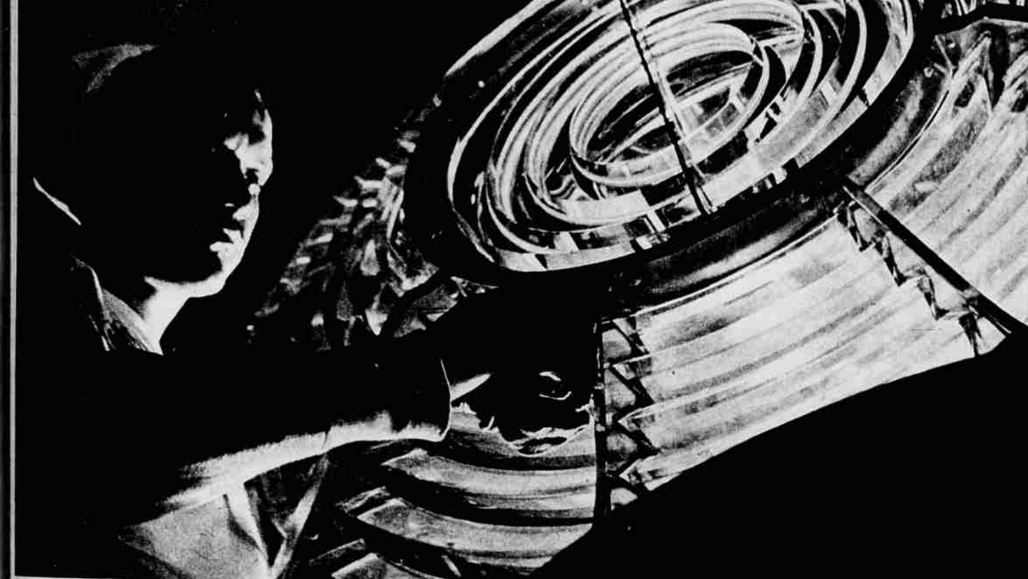
Most important job in the Montauk Point Lighthouse is the care and maintenance of the powerful beacon with its 1,000-watt lamp.
