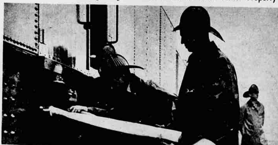
No fire hydrants here. Water or chemical is transported in tank cars. Now hoses are hooked up to kind of extinguisher best suited to type of fire.
