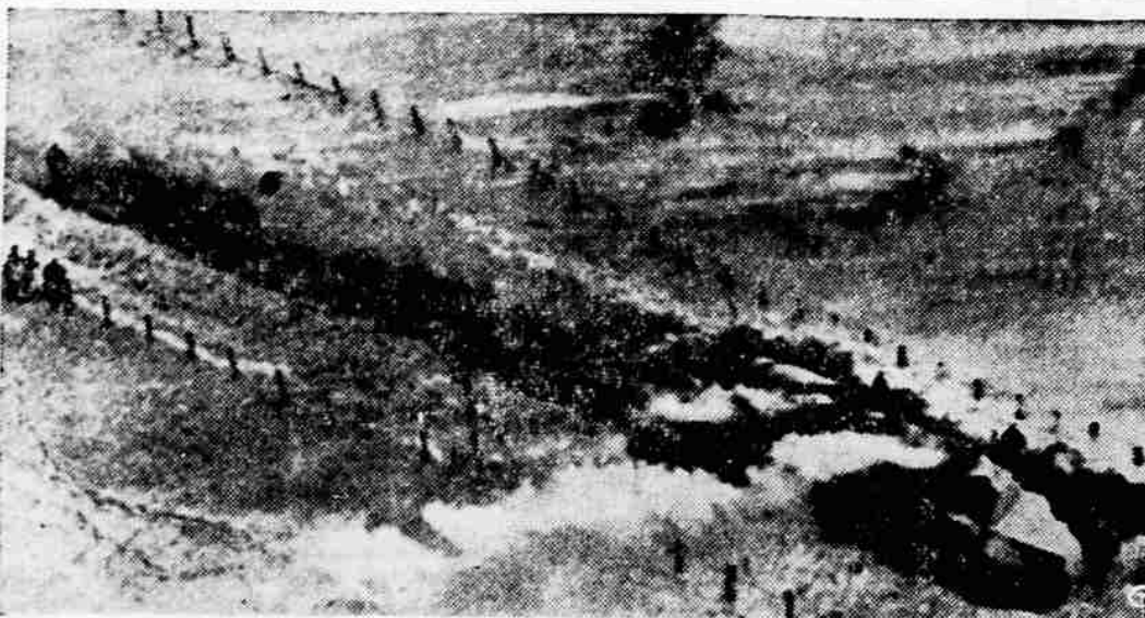
DIGGING THROUGH DEEP SNOW , workmen try to free railway engine marooned for days on Aberdeen-Peterhead line in Scotland. Unusually heavy snows have stalled traffic throughout greater part of northern Scotland for nearly a week. (International)
