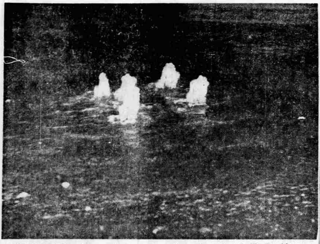
ARTESIAN WELL —As a result of recent heavy rains, Medford sewer and drainage systems were filled to capacity and in the West Main st. area the water spouted out of the holes in manhole covers. Plugged catch basins caused several intersections to be flooded and city crews were busy yesterday and today keeping the water flowing
