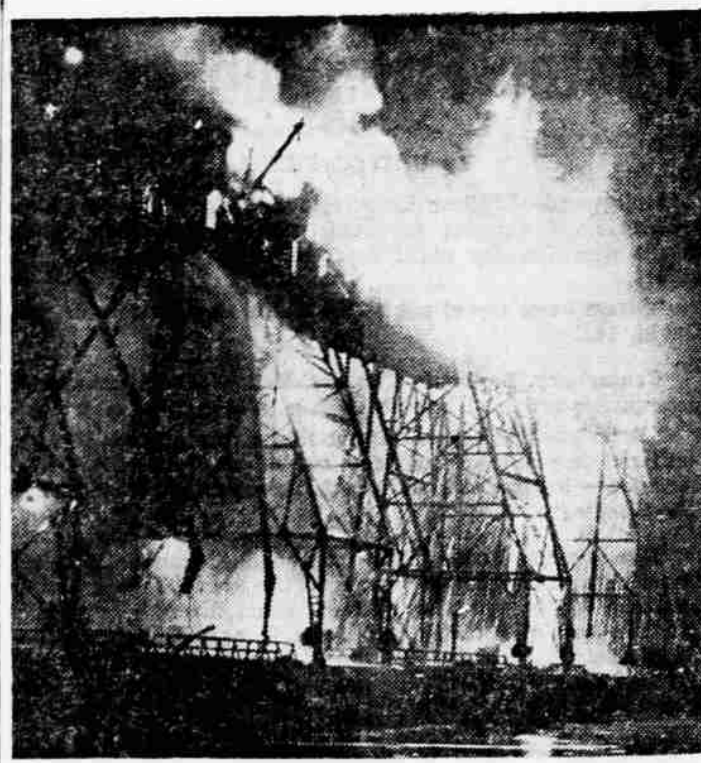
WATERFRONT INFERNO — A shower of sparks falls from grain loading dock at Vancouver, B. C., during $200,000 blaze which destroyed the structure. A Russian grain ship assisted firemen and fire boats in bringing the blaze under control.
