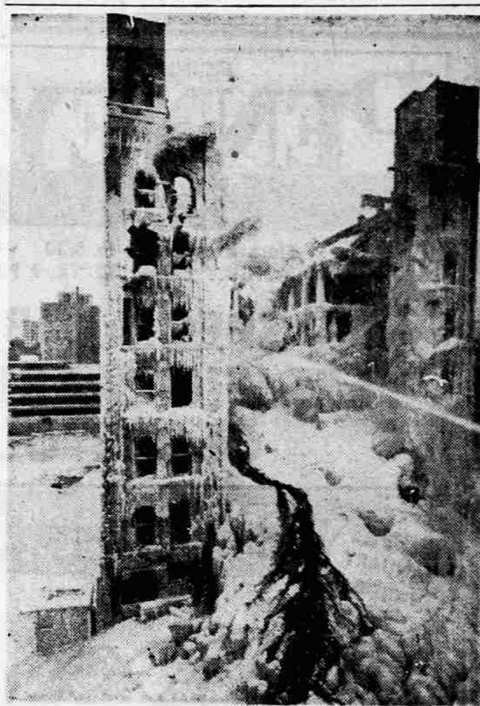
ICY MONUMENT TO PERSISTENT BLAZE —Iceicle fringes trim this bleak building in Chicago as firemen continue to spray water on its smouldering interior. Freezing temperatures and cork insulation in the walls of the building, an abandoned cold storage warehouse, hampered firefighters in their five day battle against the blaze.
