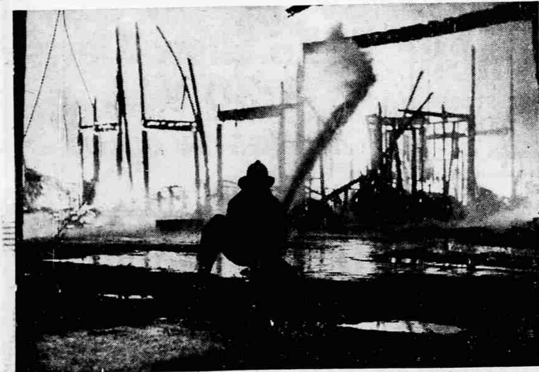
... Lumber Company Destroyed in Fire
