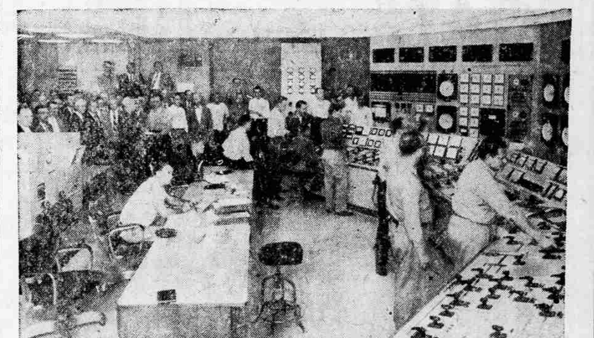
NATION'S FIRST —This is the elaborate control room at Shippingport, Pa., as the nation's first full-scale atomic power plant went into operation. Pittsburgh began to use electricity produced from the atomic power. Three operators man the controls around the clock to keep tab on the distribution system, the turbine-generator section and the nuclear reactor furnace.
