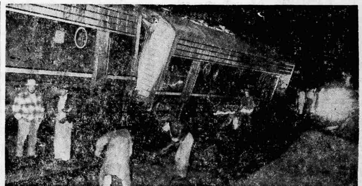
AUTO-TRAIN CRASH INJURES 16 —Railroad workers repair track near Oakley, Cal., where the crack Santa Fe streamliner Golden Gate smashed into a stalled car and derailed, injuring 16 persons. The driver of the auto, who tried to flag down the on-rushing train, was uninjured.
