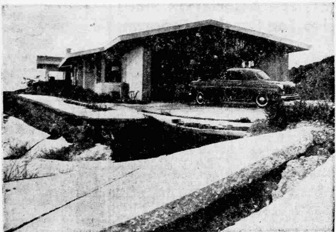
LOSING GROUND —An area known as Portuguese Bend, which faces the Pacific Ocean at Palos Verdes, Calif., has slowly been slipping away for the past two years. Here, the driveway to the home of A. W. Phillips is completely cracked up and the garage and home have started to shift. In spots the movement is as much as an inch a day. The area in the photo came in on a driveway from the right. The homes in the area are in the $25,000 to $75,000 price range.
