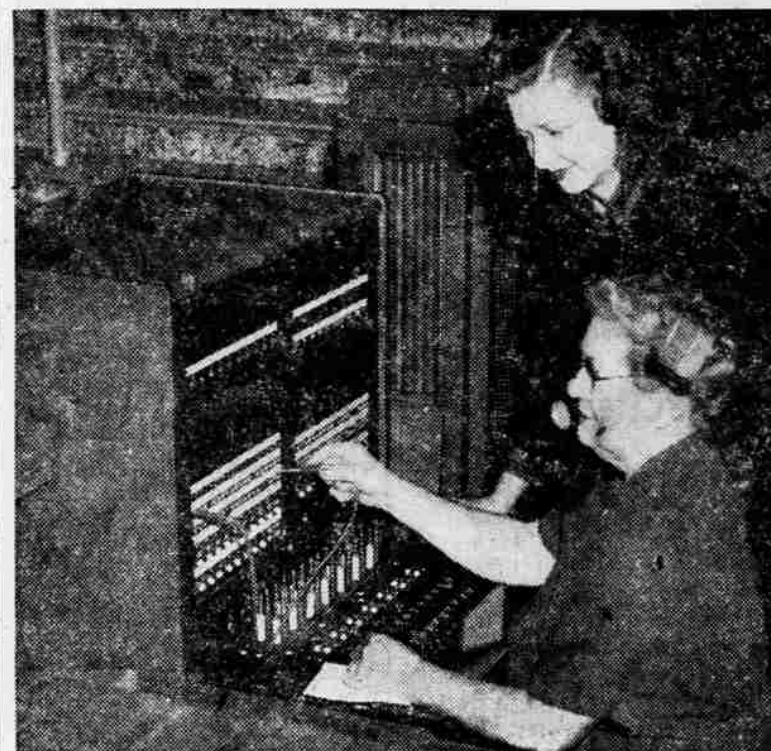
NEW SWITCHBOARD —Replacing more than 30 individual telephone numbers of the various offices at the Jackson county courthouse, this newly-installed PBX unit was put into use at 6 a.m. today, giving county offices their first centralized telephone system. Operator Mrs. Gaston Floux, seated, and Mrs. Robert Beadnel, service advisor for Pacific Telephone and Telegraph company, are shown above going over details of the operation of the new switchboard. Mrs. Floux, who is employed by the county, will also serve as courthouse receptionist. New telephone number for all county offices is SPring 3-6211. An emergency number for use after hours and on Saturdays and Sundays is SPring 3-2800.
