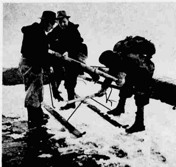
An Alpine rescue squad assembles equipment for ascent to "injured" climber in practice drill.
