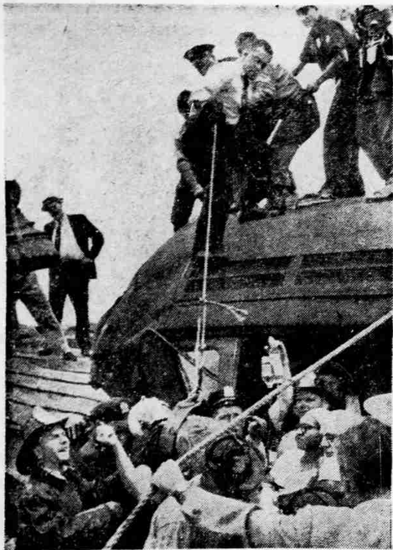
TRAINMAN EXTRICATED FROM WRECK —While an interne feeds him plasma, rescuers hoist motorman William Hochstein, 51, from the cab of one of two subway trains involved in a collision at an elevated station of the Bronx I.R.T. in New York. Hochstein, who plowed into a train standing at the station, was removed from the cab in which he was pinned for over two hours after his left foot was amputated.
