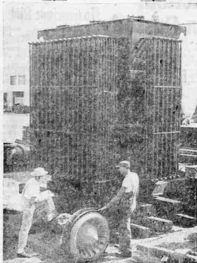
POWER PLANT EQUIPMENT —Copco employees George Bryant and Don House stand beside the 132,000 volt transformer that will soon be installed at the Eagle Point power plant now being built by Copco in the Nichols' gap area. Also pictured is the turbine that will be powered by the 435-foot head of water from an irrigation canal. The plant will operate under a constant flow of water and will provide part of the company's "base" power load.
