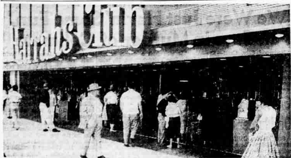
LOOK MA, NO DOORS—When Bill Harrah remodeled his club in Reno, Nev. one expense that every other building has, was left out—the cost of keys. Bill's place (above) has no doors, just a 41-foot-long air wall. Even when it is snowing on the outside, those just on the other side of the "wall" enjoy room temperature. The air wall also resists dust, insects and small animals as well as heat and cold.
