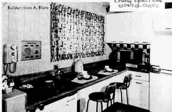
Double casement windows are set into wooden wall above Micarta counter. Note the built-in wall radio, telephone, and stainless-steel splashback.
